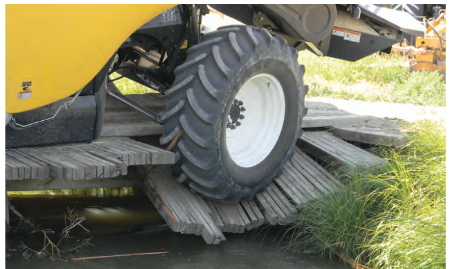
After the bridge collapsed under the front left drive tire, the rest of the combine slid in that direction, causing more of the bridge to break.
